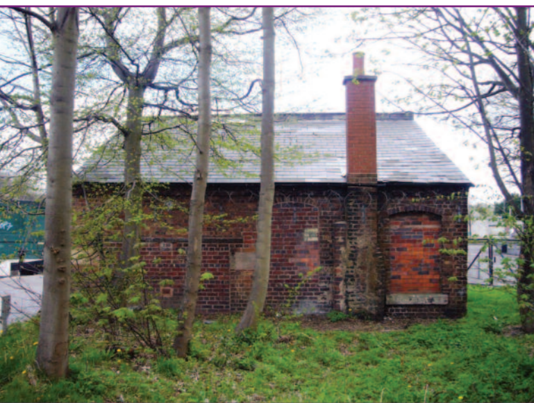
Canalside building at Stafford Road
