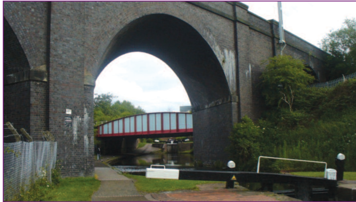
The Wolverhampton Locks Conservation Area contains a wealth of canal and railways heritage.
