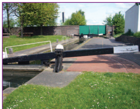
Approaching Cannock Road bridge and the green open space at Lock 5.
