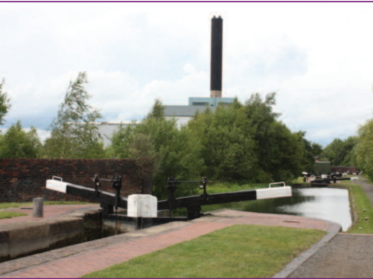
View north from Lock No. 6 with the Wolverhampton Municipal Incinerator in the distance and the sites of the former Crown Galvanising Works and Ceres Works to the left.
