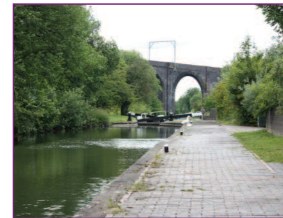
View towards the Oxley Viaduct from Stafford Road Bridge.
