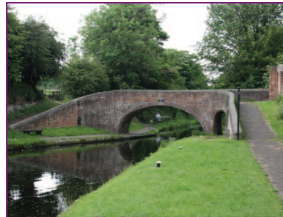
The grade II listed bridge over the Staffordshire and Worcestershire Canal is an excellent example of a roving bridge built to allow the boat man and his horse to cross the canal without having to uncouple the hauling line from the boat.
