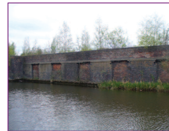
The canalside wall of the Ceres Works covered loading bays.
