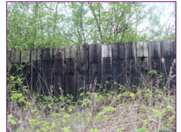
A fence of reused railway sleepers just south of Cannock Road enclose the towpath and mark the former site of Cannock Junction
