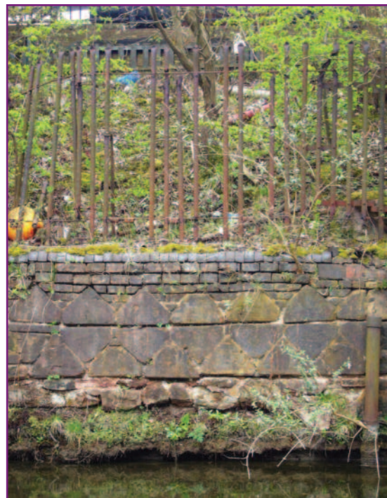
Spike Island fencing on top of a wall constructed using wall copings giving a 'dog's tooth' effect facing the canal.
