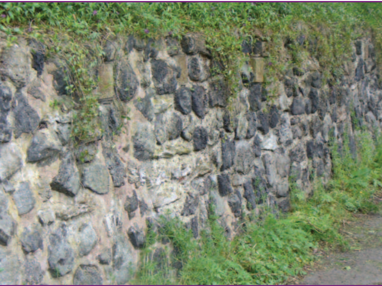
A locally distinctive wall of foundry slag near Fox's Lane bridge
