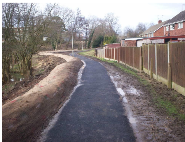
Figure 3 - Defence bund and wall installed adjacent to the River Stour at Grange Crescent, Halesowen in 2012, in partnership with the Environment Agency
