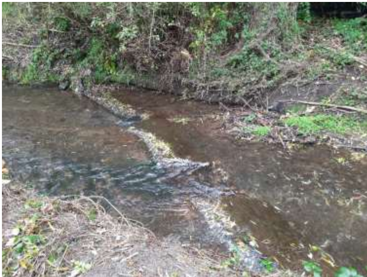
Figure 75 - Weir upstream of the reedbed, proposed for removal
