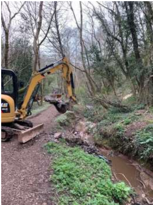
Figure 80 - Work in progress on removal of two of the weirs.
