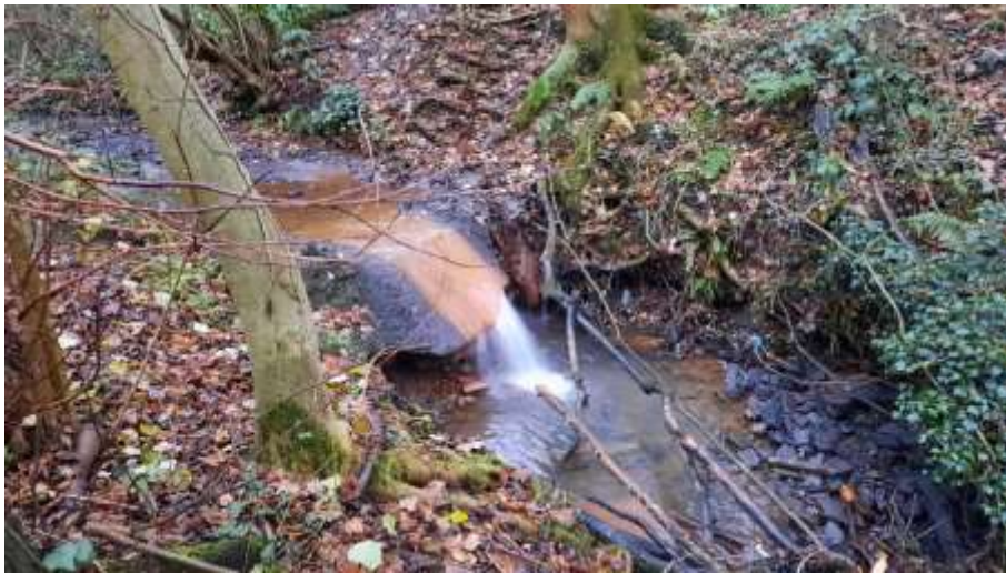
Figure 79 - Despite undercutting, this weir is a major barrier to fish passage.
