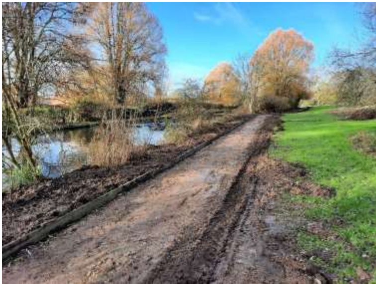
Figure 13 - Path cleared and side boards fitted ready for resurfacing.
