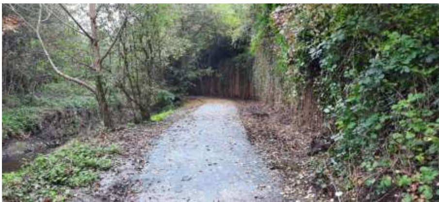
Figure 65 - In a change to the original proposals, a bound gravel path was chosen over a boardwalk
