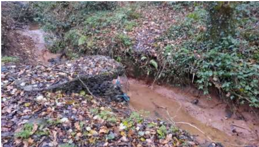
Figure 78 - Almost completely broken up weir.
