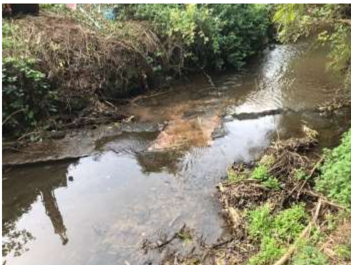
Figure 76 - The weir with central portion removed and (right) riffles created upstream as a result of removal.
