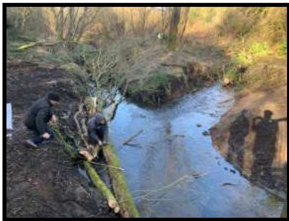
Figure 73 - Steel wire leashing on chop and drop in line with specifications outlined within the Ordinary Water Course consent. With the bund in place the greater flow can be seen on the lefthand channel.
