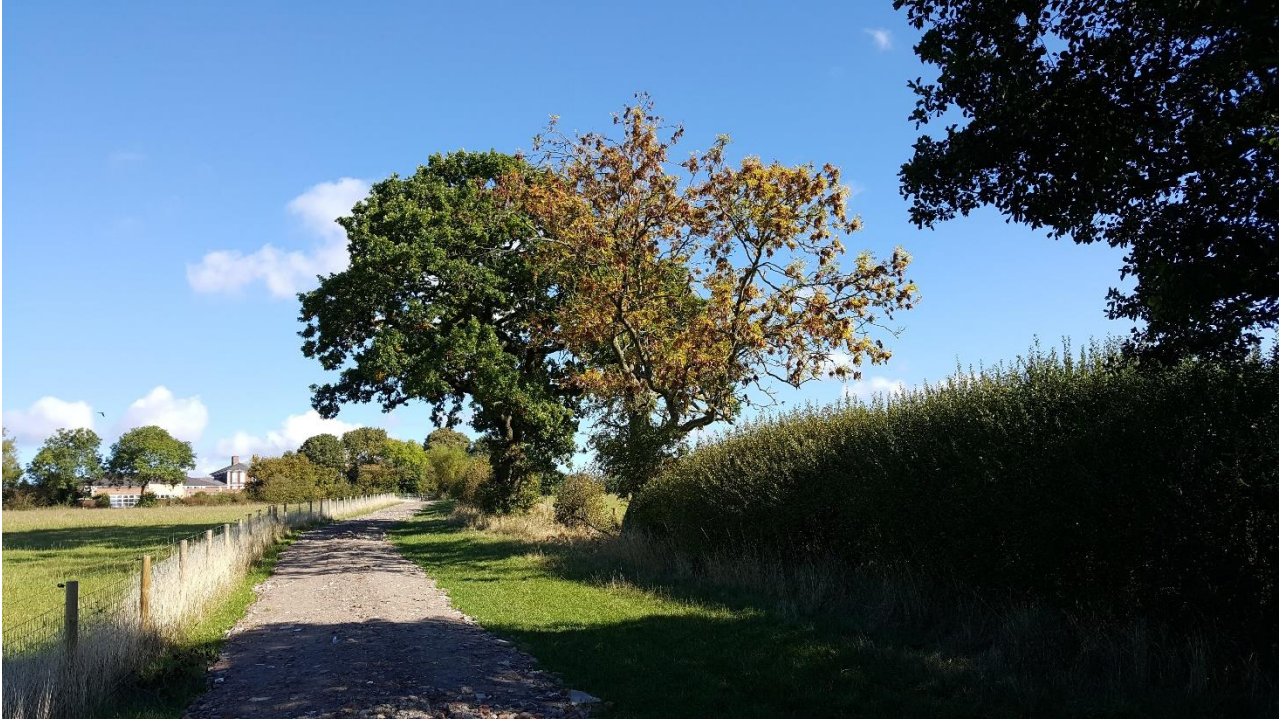
Recently layed access track of crushed recycled demolition material adjacent to hedgerow 7.
