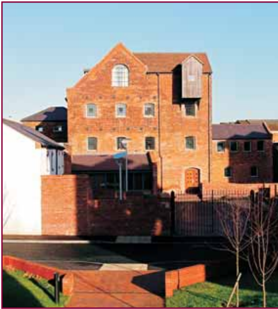
Above: The recently refurbished Albion Mill.
