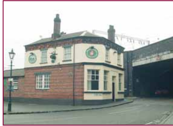
Above: The Great Western public House and Corn Hill Railway Bridge
