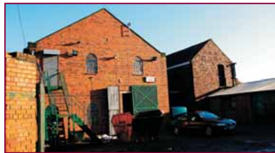
Above: Union Mill buildings
