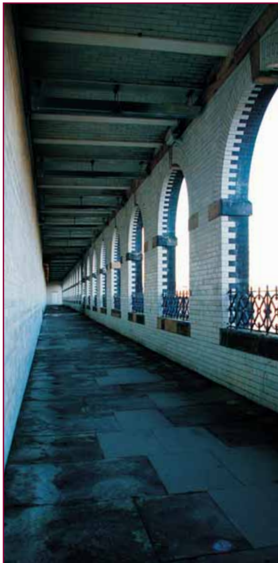
Above: Pedestrian gallery and underpass link between high and low level stations. 'The Colonnade'.
