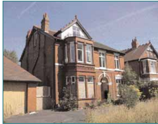
Above: Vacant properties in Albert Road
