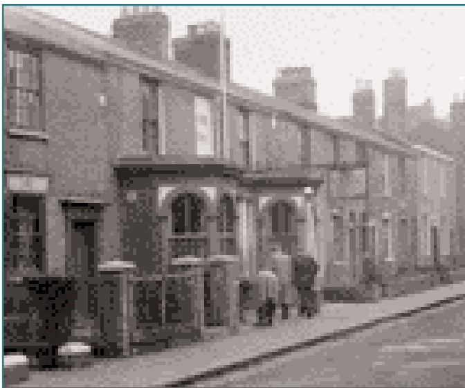
Above: The Vine Inn, Lower Vauxhall was one of many buildings demolished for high rise developments in the 1960s.
