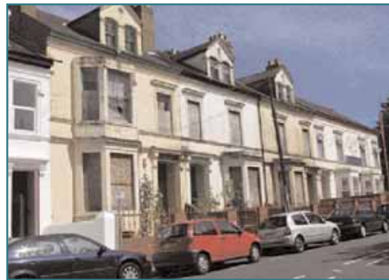
Above: Boarded up properties in New Hampton Road East and Sikh Temple far right.
