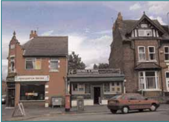
Above: 243 New Hampton Road East
