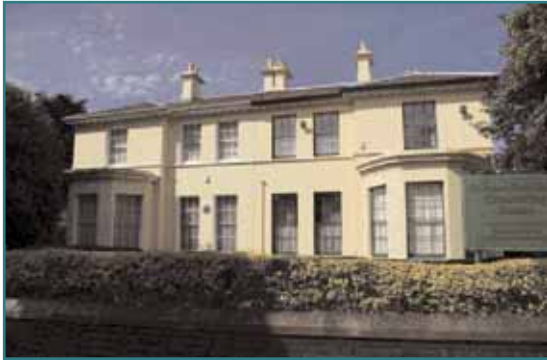
Above: Grade II Listed Nos. 7 & 8 Summerfield Road
