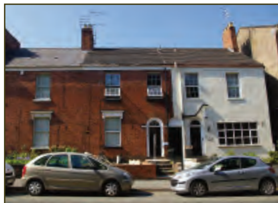
Unsympathetic alterations are a threat to the character of the conservation area.
