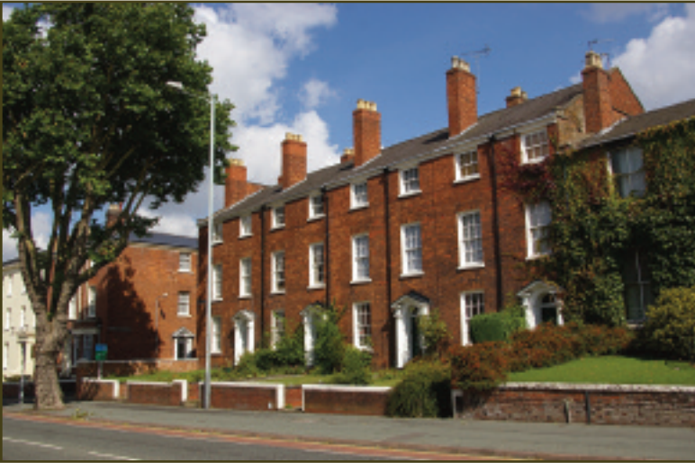
Green frontage to Nos 24 – 32 Tettenhall Road.
