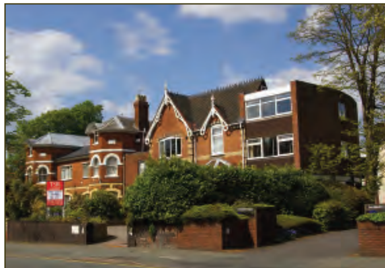
Insensitive extensions to historic buildings have a negative affect on the character of the conservation area.
