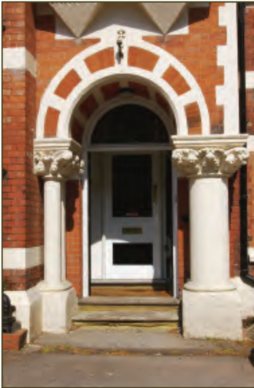
The porch at Berrington Lodge.
