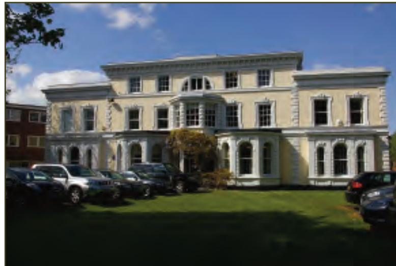
Grade II Listed Building Salisbury House.
