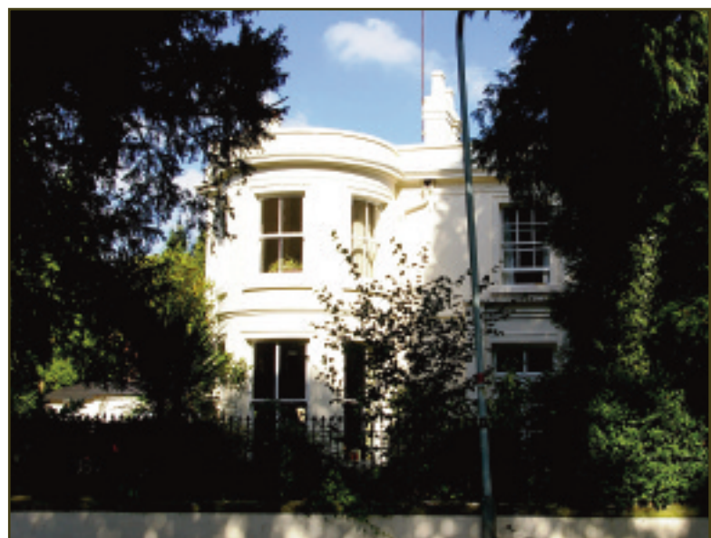
Crescent House, Locally Listed building.
