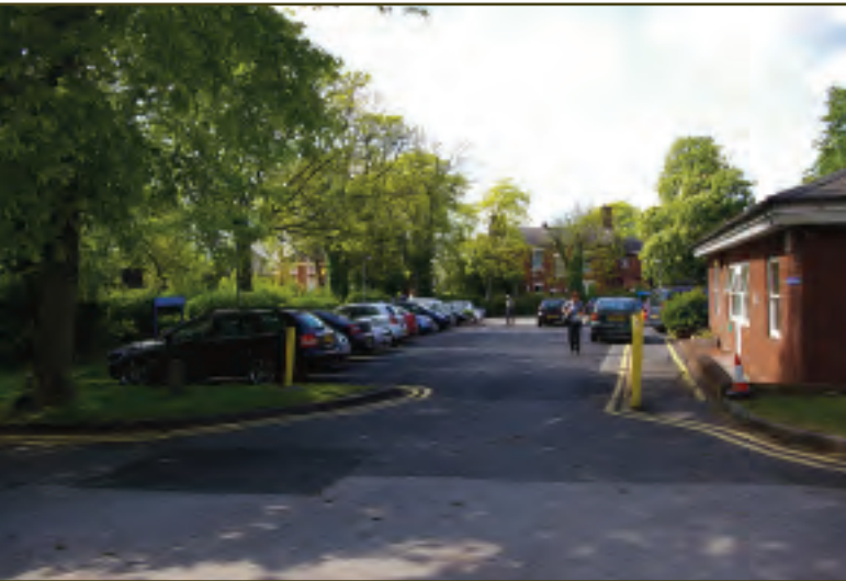
Modern hospital buildings and car park at the junction with Connaught Road.
