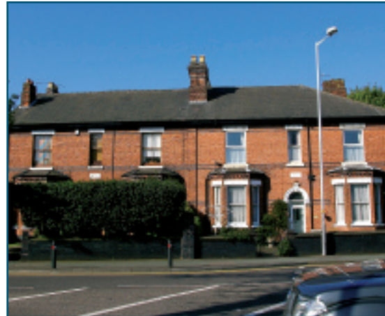
Above: Large brick semi-detached houses Stubbs Road
