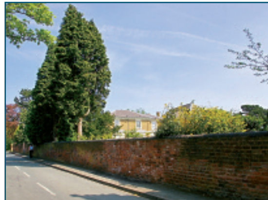
Above: Boundary Wall in Poplar Road
