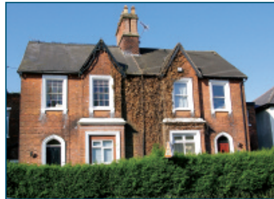
Above: Unsympathetic alterations erode special character
