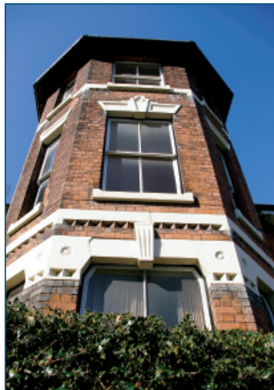
Above: Canted bay at 29 Stubbs Road
