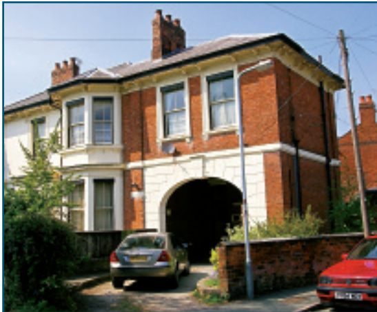
Above: Porte-cochere at 38 Riley Crescent
