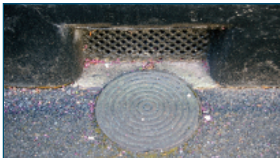
Above: Coalhole cover in Chequer Street
