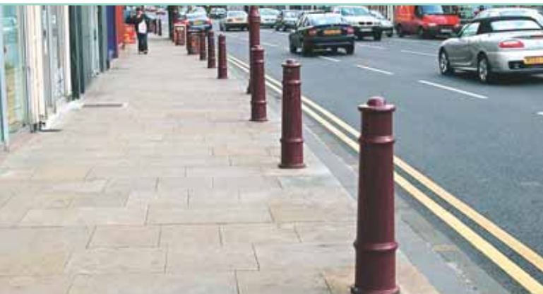
Above left: Natural stone paving, Chapel Ash (north side)
