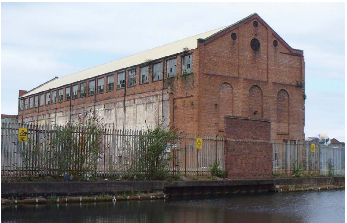
The turbine hall of the former power station on Commercial Road
