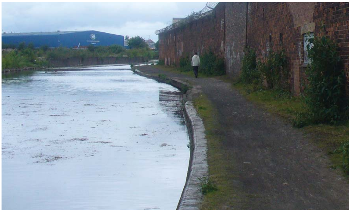
Towpath near Cable Street with beaten gravel path with canal bank materials including concrete (marking the entrance to a former basin), bull-nosed blue brick and iron rails adding extra support to the bank.
