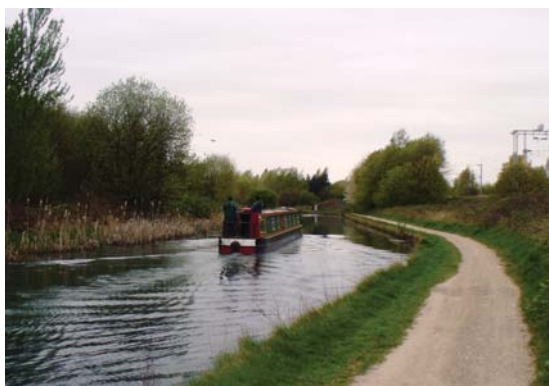
The winding course of the canal was designed to follow the contours of the land.
