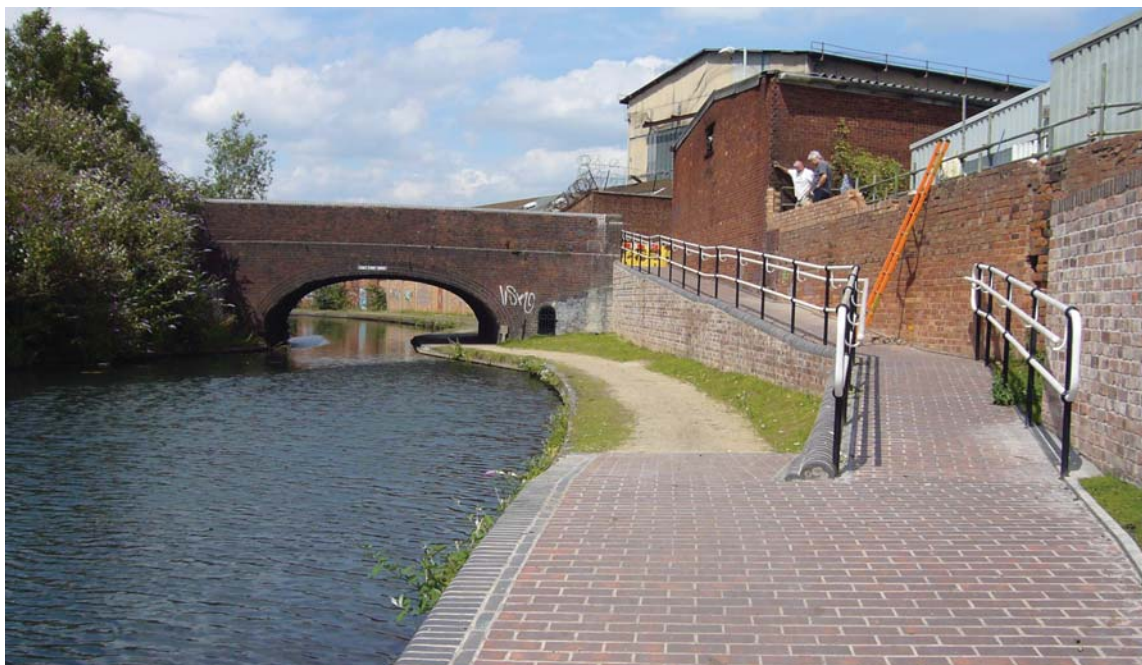
Cable Street Bridge was built in the mid 19th century. Recent towpath and access enhancements were undertaken under the ABCD New Deal for Communities initiative.
