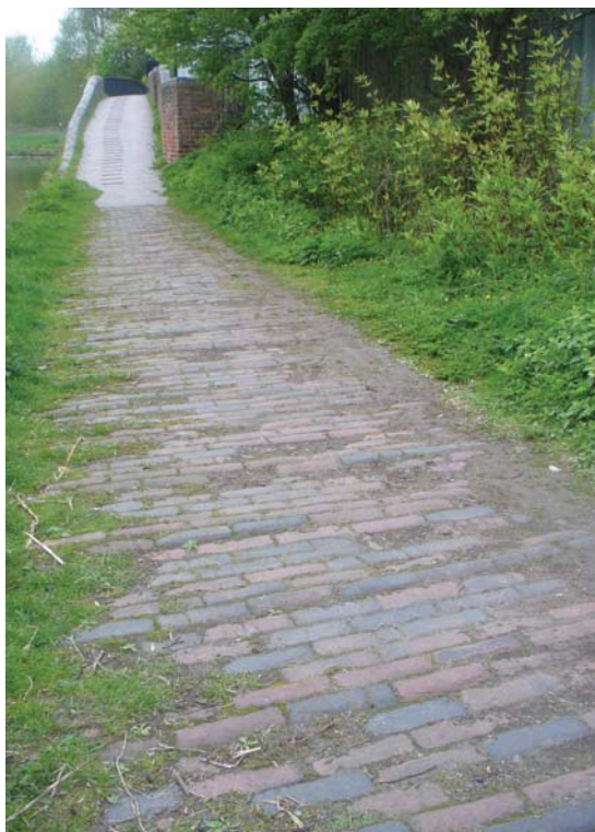
Brick paving on the approach to Deepfields Junction Bridge.
