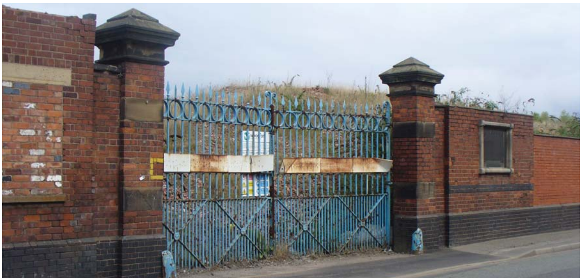
Caption: Historic boundary treatments at the former Monmoor Ironworks, Cable Street.
