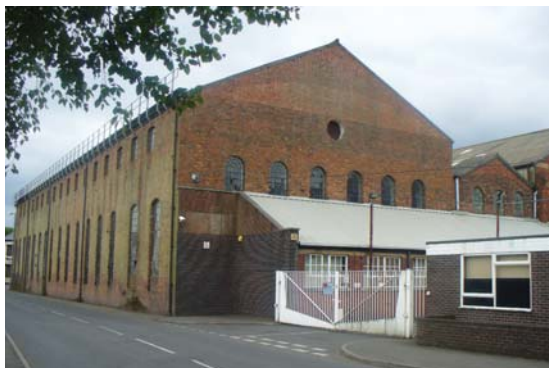
The Highfields Ironworks building which is a significant landmark building and a rare survivor.
