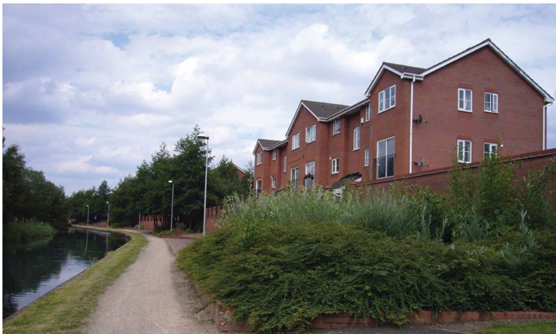
The canalside at the Millfields development.
