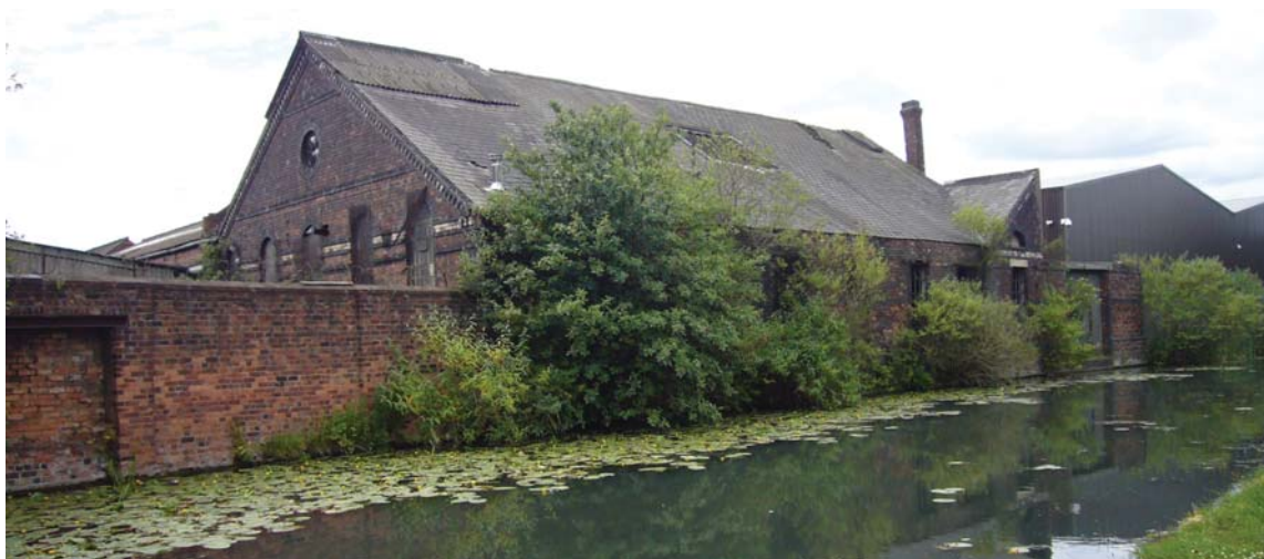
Remains of the New Griffin Works with its distinctive polychrome brickwork and cast iron windows.
