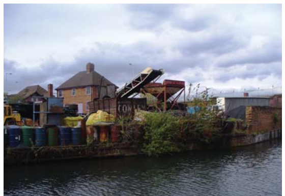
The Wulfruna Coal Company at Minerva Wharf preserves the character of a working coal wharf.
