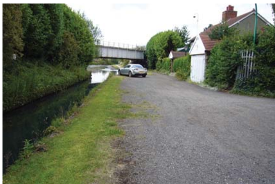
Stop-Lock chamber between Ettingshall Road and Dixon Street with the railway bridge behind and altered canalside cottages possibly once associated with the management of the lock.
