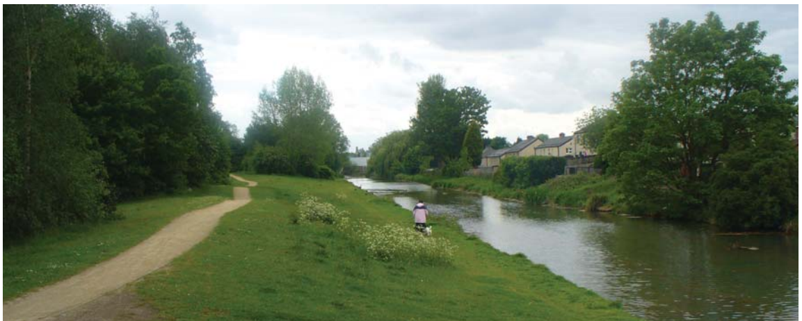
The Bradley Arm is kept open due to its role supplying water to the wider network and to provide access to the Canal and River Trust Depot.
