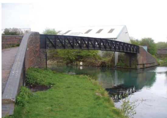
The iron towpath bridge at Deepfields Junction.
