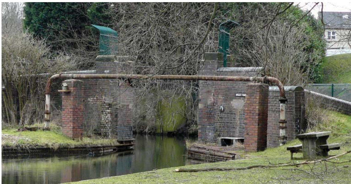
Surviving former towpath abutments at the Canal and River Trust Depot. The basin here is all that remains of the old route, that ran between here and Loxdale sidings. The current straight stretch of canal dates from improvements made in 1817.
