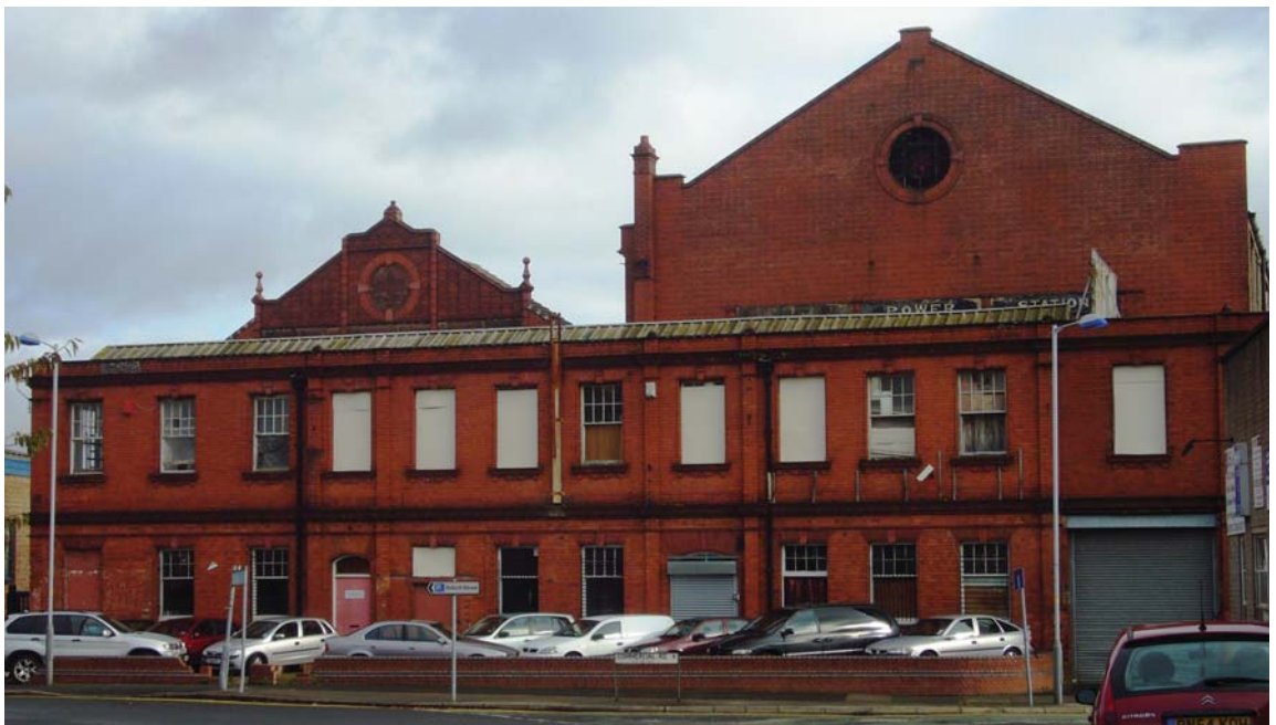
View of the 19th century power station in Commercial Road.
