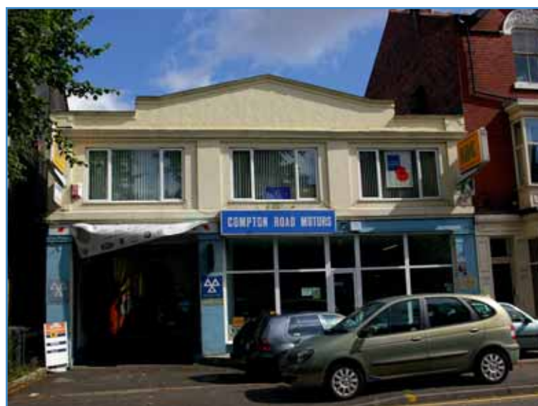
Above: 1930s car showroom on Compton Road
