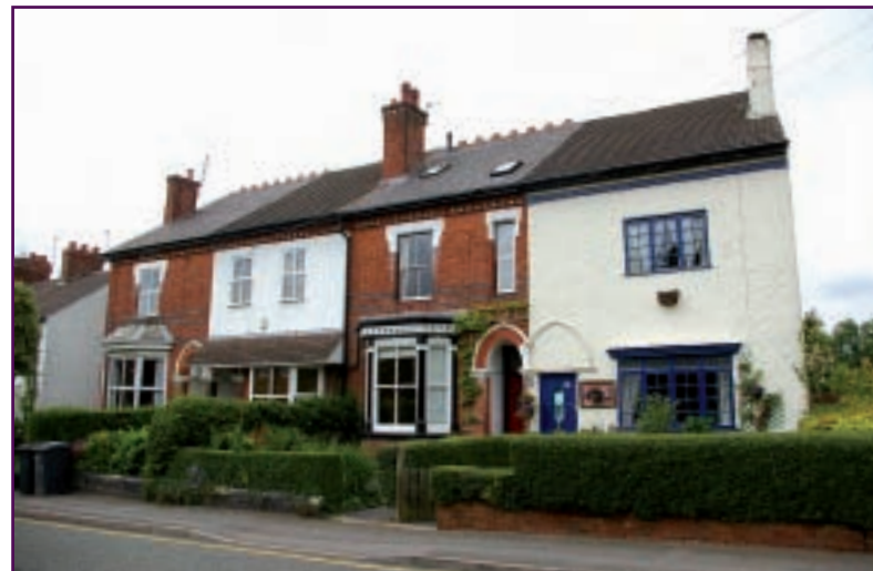
Above: Incremental changes can damage local character
