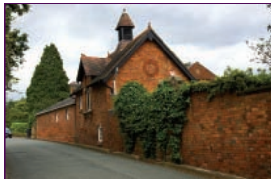
Above: Brick boundary walls and converted coach-house, Ormes Lane.
