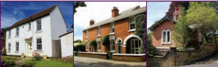
Far left: 22 Ormes Lane Middle: 26 - 28 Wood Road Left: The Lodge, The Holloway
