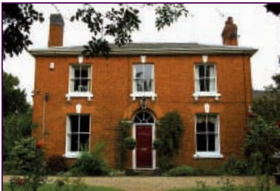
Above: No 1 Church Road
