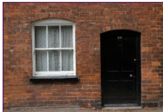
Above: Detail of cottages in Wood Road
