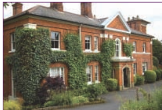
Above: Bromley House, Ormes Lane
