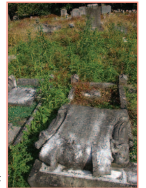
Above: Damaged churchyard monument
