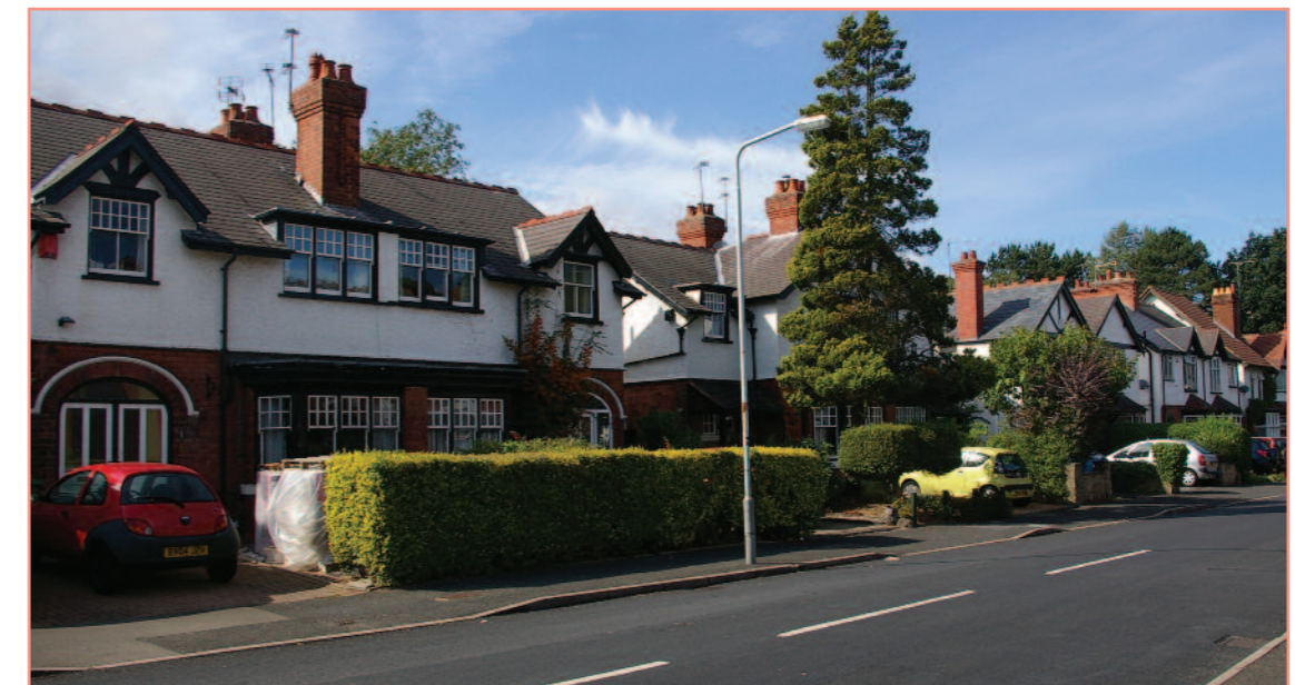
Above: West side of Church Road
