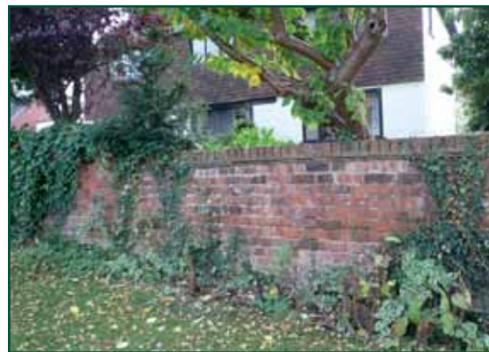
Above: Front boundary wall at No 26
