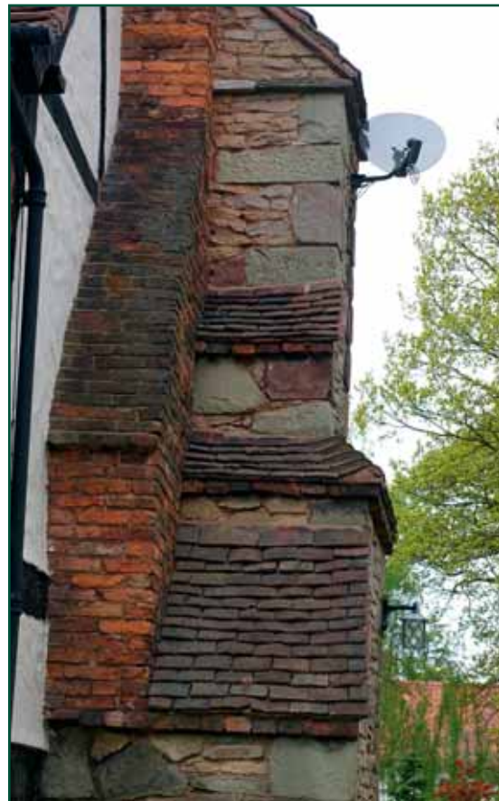
Above: Reclaimed stone used in the chimney of No 36.
