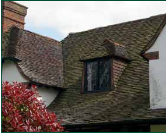
Above: Sweeping clay tiled roof and dormer window.
