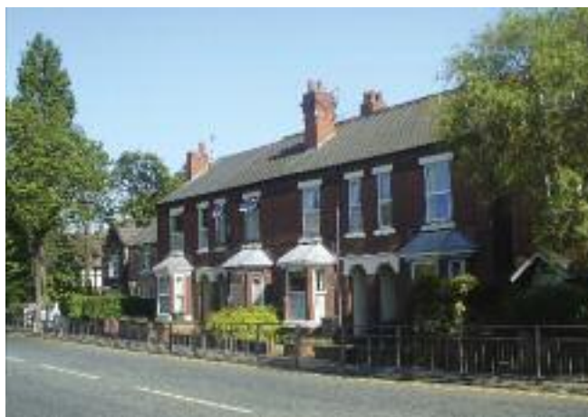
Houses in Mount Pleasant are now protected by the Article 4(1) Direction.
