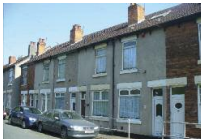
The character of many of the houses in Lewis Street has been eroded through loss of attractive original architectural features.
