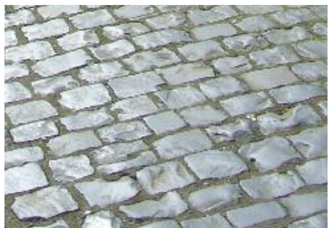
Local Rowley Rag dolerite paving at 24 Lichfield Street
