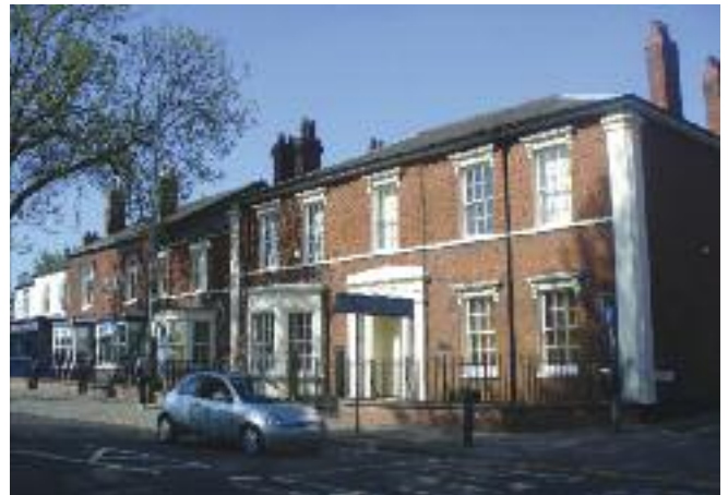
Late Georgian townhouses on Wellington Road. No 3 Waterloo House is Grade II Listed.
